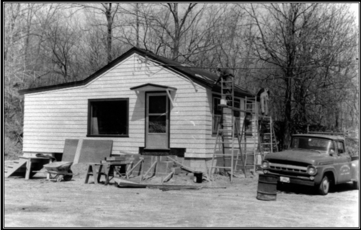
Originally a flower shop on Wellington Avenue, this building was moved to the range to be used as a classroom around 1964. (Black & white photo's courtesy of Sgt. William Loux – CPD retired)
